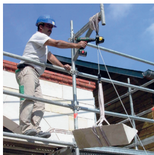
Sollevamento carichi. Lifting loads.
